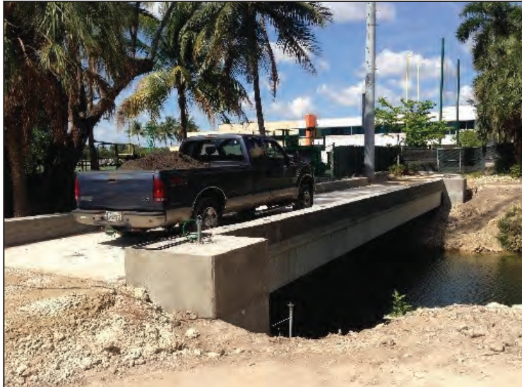
Figure 4. Load testing with pick-up truck
