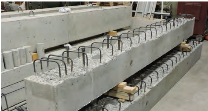
Figure 1: Casting of two sets of partial beams, three beams per set
