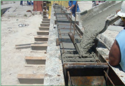
Figure 1: Left: casting of beam 3. Right: beam 5 with three sets of prestress strands
