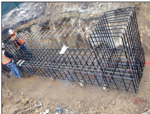
Figure 3. Reinforcement cage for pile cap, side blocks and back-wall
