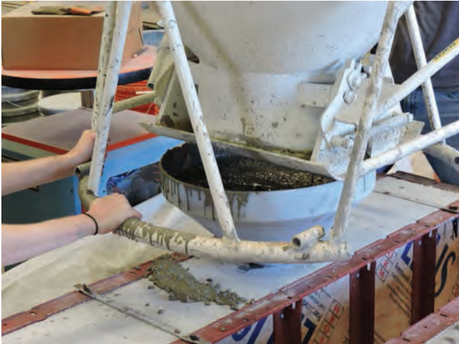
Figure 4. Repair Material Placement
