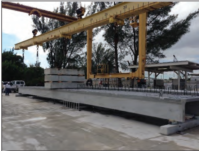
Figure 2. Double-tee static load test at precast yard
